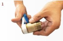
(A) Pipe side: Apply PTFE thread seal tape or pipe joint compound to the tapered threads of the inlet nipple.(B) Flexible hose side: DO NOT use both pipe PTFE or pipe joint compound
