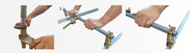
Connect the nut of the flexible hose to the outlet reducer. DO NOT use PTFE or pipe joint compound since on outlet reducer at the hose side since there is already a seal gasket in place to seal the joint. Tighten the
