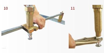
With outlet reducer positioned inside the center bracket, grasp and firmly close the handle completely to secure the reducer in place. Apply PTFE or pipe joint compound to the male threads of sprinkler. Install the sprinkler into the female threads of the outlet reducer by following sprinkler manufacturer's installation instructions.
